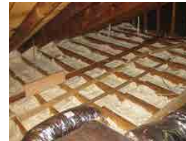
During monolithic coating of entire attic floor (1" of foam)
