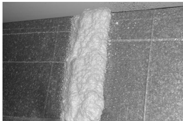
FIGURE 1—DUCT JOINT SEALING
