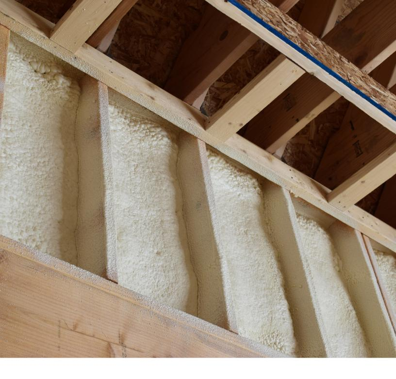
ICP Building Solution Group's HVLP foam technology developed with a leading systems house and Spray Foam Systems, the leader in HVLP dispensing equipment, performed extensive testing and technical development to provide a perfect foam and dispensing solution for high volume, low pressure applications.
