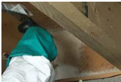
Ideal for flash and batt or hybrid insulation systems or in applications where a Class 1(A) and Class 2(B) material is required. Stops air infiltration and provides an aged R-value of 6.1 at one inch thickness for an economical, efficient insulation system.
