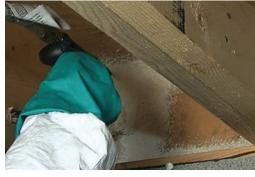
Ideal for flash and batt or hybrid insulation systems or in applications where a Class 1(A) and Class 2(B) material is required. Stops air infiltration and provides an aged R-value of 6.0 at one inch thickness for an economical, efficient insulation system.
